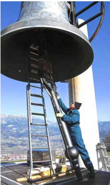
23 March, 2016: The new Maria Dolens clapper made by the Capanni company is positioned
